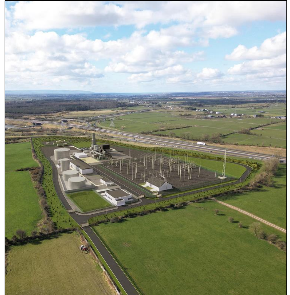
(Source: Bord Gáis Energy Ltd showing Cashla Peaker Plant)
